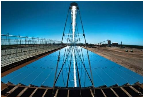
[Areva](#)'s solar unit consisted of what remained of the acquired startup [Ausra](#) and its compact linear Fresnel reflector (CLFR) solar steam generator technology.
